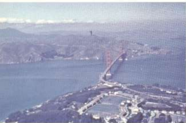
San Francisco Golden Gate Bridge
